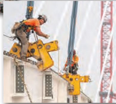
Workers prepare a floor beam to be erected into the bridge deck for the Gordie Howe International Bridge. Each floor beam weighs 55,115 pounds and measures 113 feet in length. (Photos Courtesy of WDBA)
