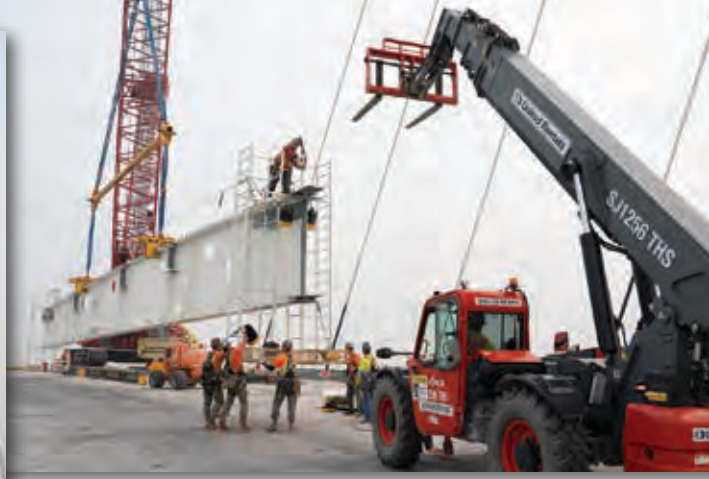
Workers prepare a floor beam to be erected into the bridge deck for the Gordie Howe International Bridge. Each floor beam weighs 55,115 pounds and measures 113 feet in length. (Photos Courtesy of WDBA)
